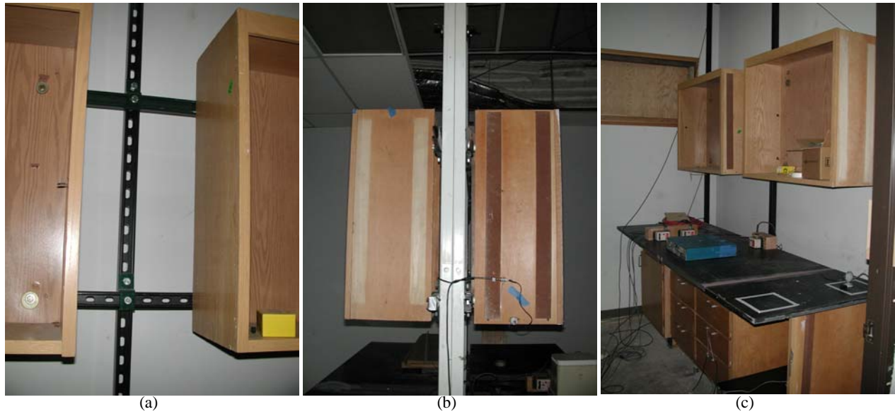
Figure 4. Typical bench-shelf details: (a) horizontal-vertical connections, (b) back-to-back, and (c) single bench-shelf systems.
